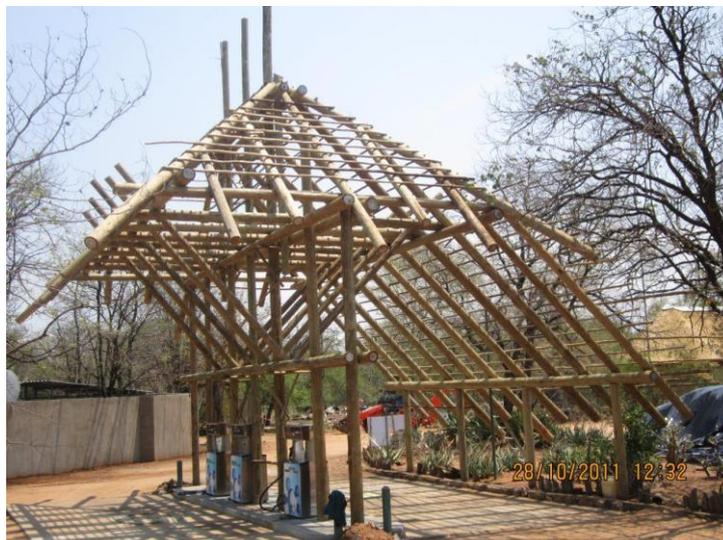
This structure is built from CCA treated Sydney blue gum. The timbers were lightly sanded and coated with a brown wood sealer. The roof is low down on one side to keep out the afternoon sun and the front open to allow easy access to the bowsers.
