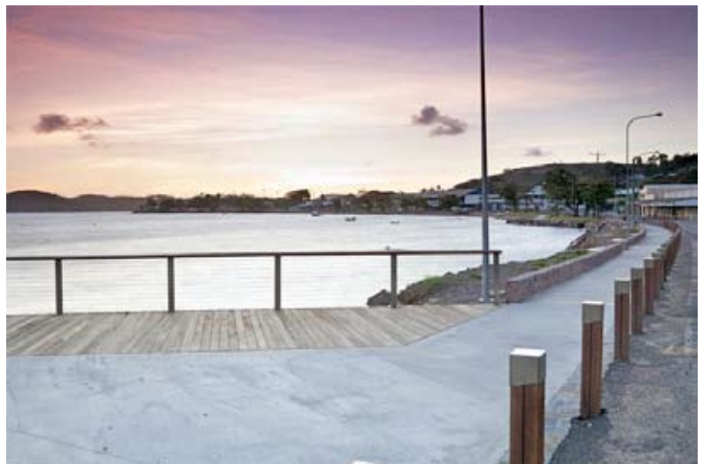
150x150 bollards used successfully on Thursday Island as detailed by OSA
