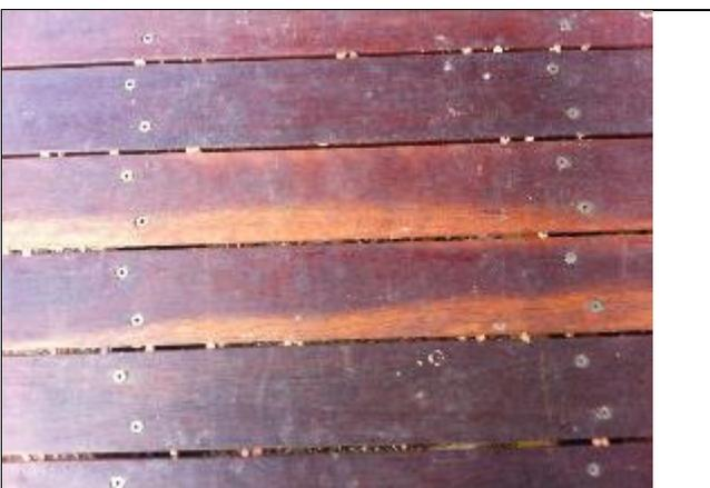
Figure 2. Untreated sapwood on face
