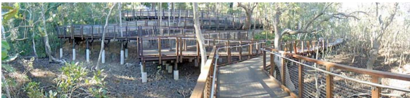
The scope of works comprised two parts. The first, to construct a new access ramp from the lower car park, leading up to the entrance of the wildlife sanctuary. An elevation of approximately 9.5 metres with 153 lineal metres of timber decking and switchbacks.
