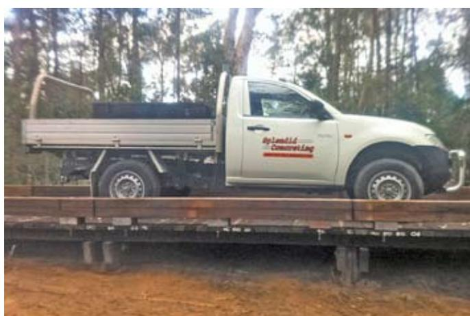
This boardwalk was unusual in that it needed to carry a 2.5tonne, 4 wheel drive fire vehicle. We prepared the drawings for the superstructure based on our standard systems and then emailed the AutoCAD drawing through to the engineer. He checked them and simply dropped the file into his drawings and then designed the site specific superstructure. With OSA preparing the layout the many points of detail we incorporate into our boardwalks were fully detailed.
