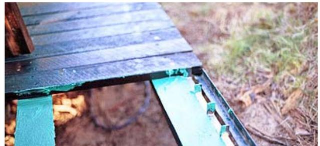
Boardwalk by OSA with Malthoid on top of joists and CN emulsion on top of the Malthoid
