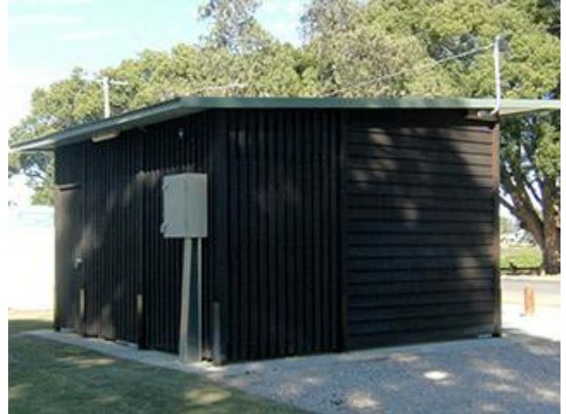
Large storage area at back of toilet
