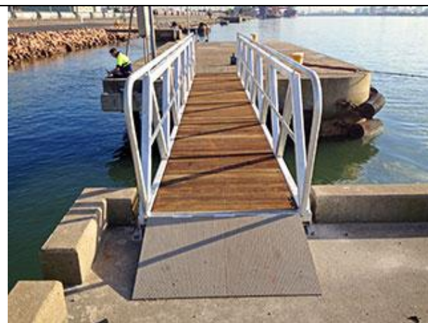
Gangways built by DWW with Infrastrucxion Deckwood
