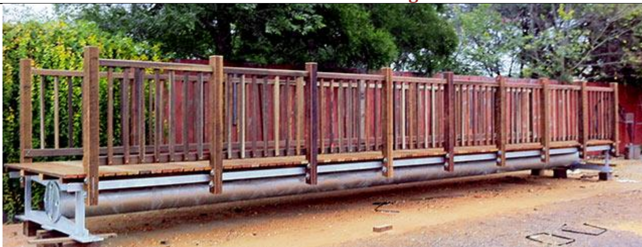
Somerset bridge with Queensland handrail ready for dispatch
