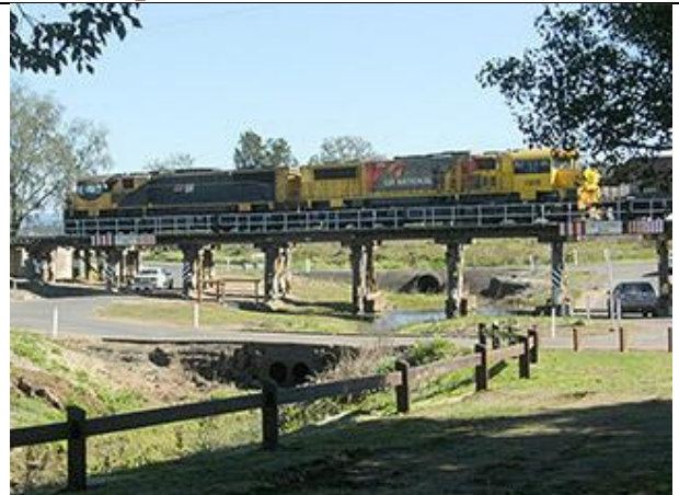
The Grantham railway bridge now with Infrastrucxion Std heavy duty traffic barrier and bollards in foreground
