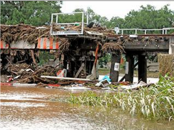
The Grantham railway bridge after the flood, image courtesy of Bruce Horrocks of the Gatton Star
