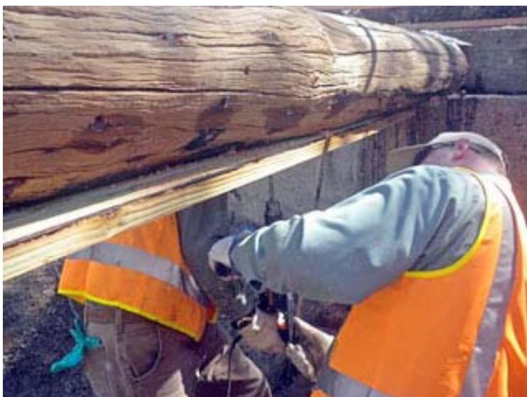
Retrofit by chemically welding Kevlar to a log stringer
