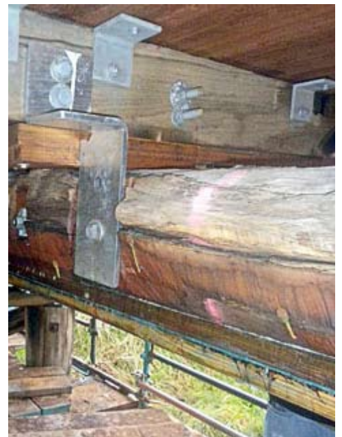
Horizontal bolting, diffusing and injected log stringer
