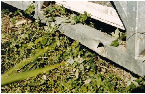
Thin steel damaged by mower
