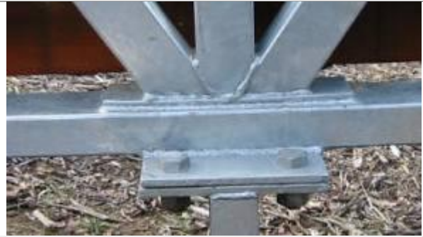
Thin steel needs stiffener to attach braces
