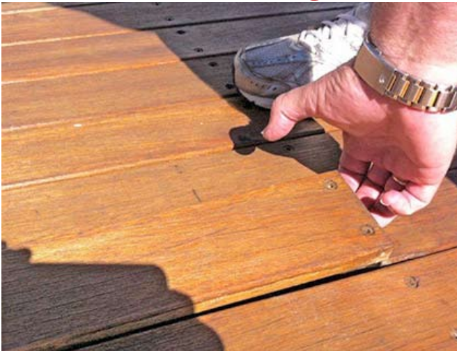
Fixings breaking in C section steel
