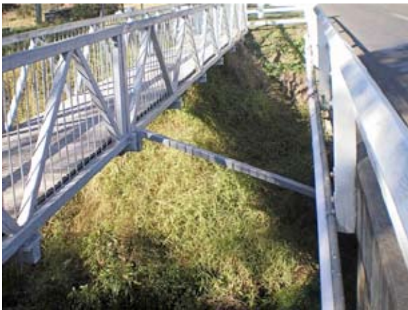
Unsuitable bridge needed bracing back to existing road bridge
