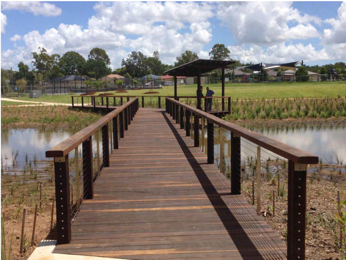
Site address, Pioneer Park Harley St at Shailer Park
