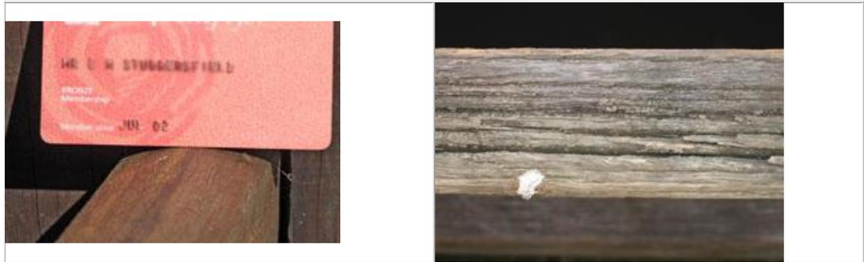
One thing we noticed is the need to shed moisture on these rails even though they only have a small top surface area. The rail on the right is a 20 year old piece from one of my bridges. I thought, I could do better and after taking that image always ensured that the tops of our rails had a radiused top surface. Not enough years have gone by to tell you it is a great success but it should perform better.
