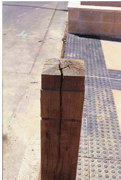
The images above are from a project OSA refused to supply as the specification was inadequate. We would have only supplied them with a metal cap and an expansion groove down the length. The client, as often happens, took the lower price option and now the bollards are badly torn down the length and top with gaps so big that children can catch their fingers. OSA has now supplied the client with a metal cap fitted but the unsightly tear remains.
