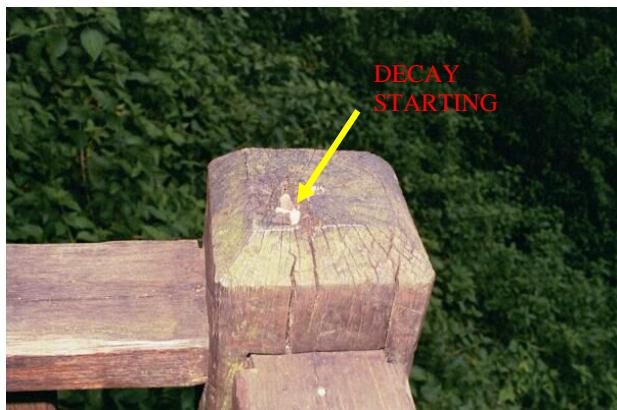
The post on the left is 150x150 with the heart in the centre. Because the heart is much softer than the surrounding true wood, the centre decays as the image shows. A metal cap protects this soft timber from decay and also restrains the top and helps minimise the splitting.
