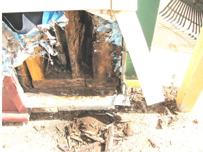
Part of the corner studs can be seen at the bottom
